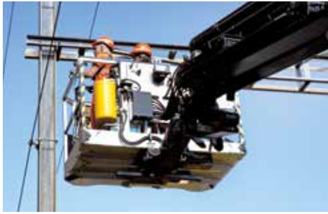
WORKMAN BASKETS FOR WORKING ON OVERHEAD WIRING
