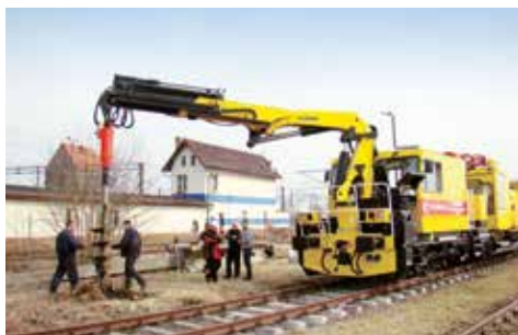
AUGERS TO PREPARE MAST FOUNDATION HOLES
