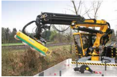
BRANCH SAWS TO CUT THE STRUCTURAL CLEARANCE OUTLINE ALONG THE LINE
