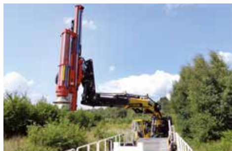
PILE DRIVERS TO DRIVE MAST FOUNDATIONS INTO POSITION
