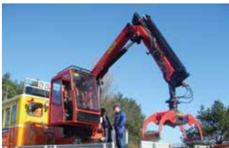
TIMBER GRABS TO POSITION SLEEPERS AND RAILWAY ELEMENTS
