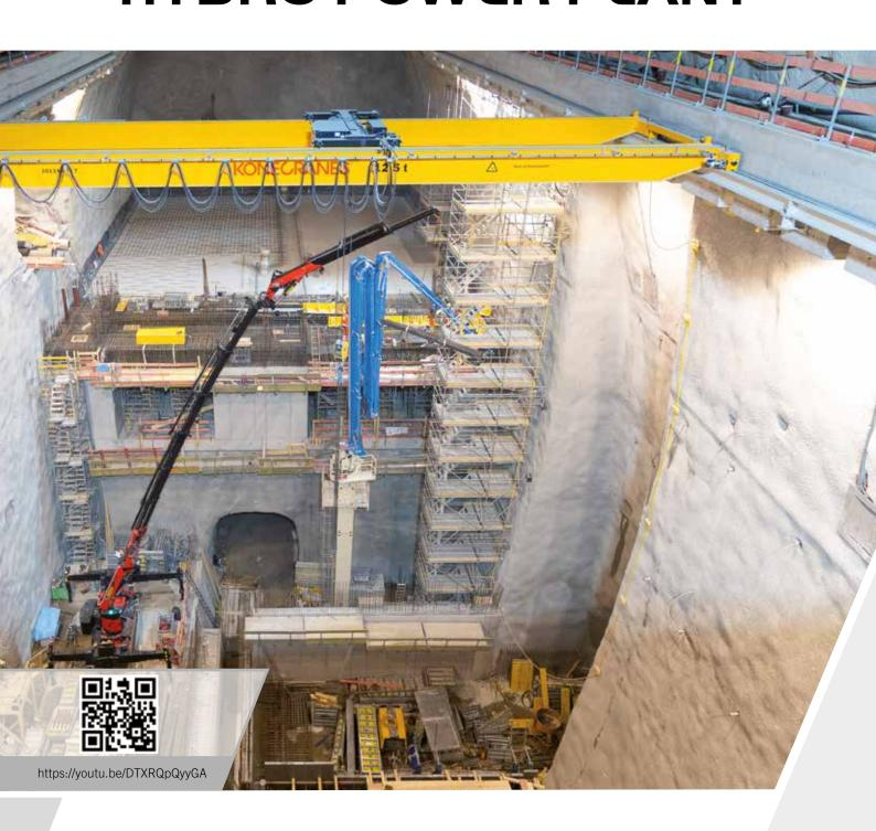
Compact and agile, strong and stable - the PALFINGER PCC 57,002 crawler crane lifts even the heaviest construction components on site with ease and precision. The environment and the construction workers inside the cavern benefit from the emission-free and silent operation of the compact crane.
