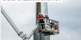
Working on telecommunication masts and on power lines requires particularly strong safety features. Overhead lines, for instance, must be disconnected if the work platform is not strongly insulated. For live power lines up to 1000 V, a double-insulated basket already provides excellent protection.
