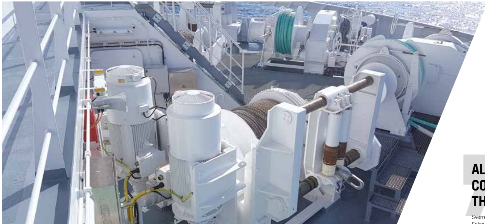
6-point mooring system winches
