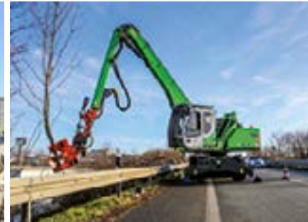
S5 – Excavators / wheel loaders
