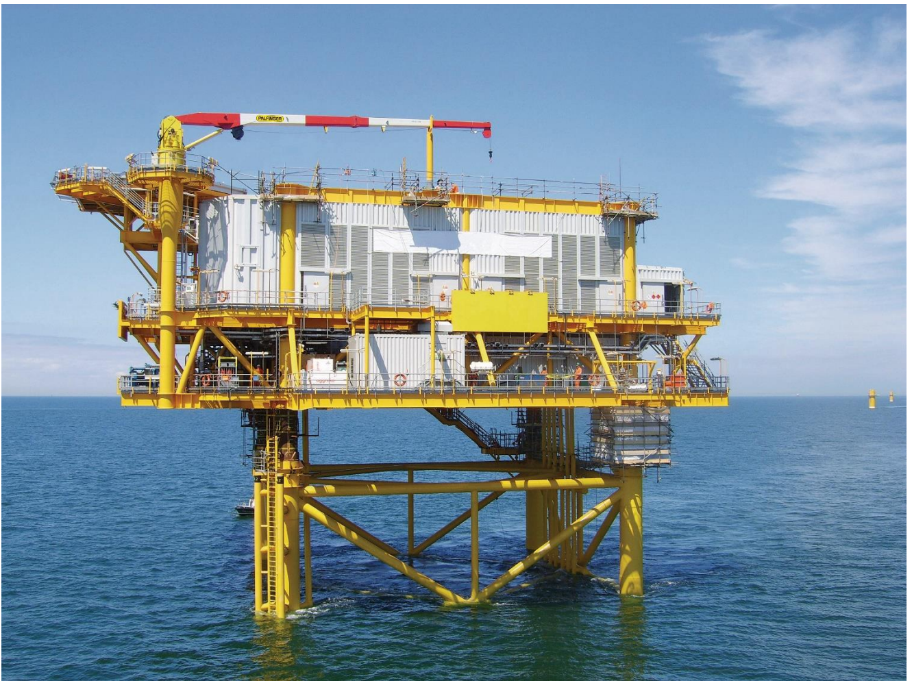
Image of a PALFINGER MARINE stiff boom crane installed on an offshore substation. © PALFINGER
