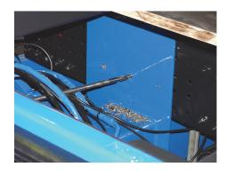
➤ Drill the holes in the console plates. The hole pattern of the bearer can be used for this. If there is no hole pattern on the bearer, the bearer must be drilled through.
